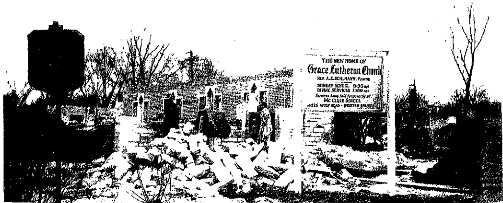
The new church building in progress. A Cornerstone Laying Service was held March 23, 1952. It is on the northwest corner of the church dated 1952 and contains a metal box holding a Bible, church papers, list of names of members and Sunday School students.
